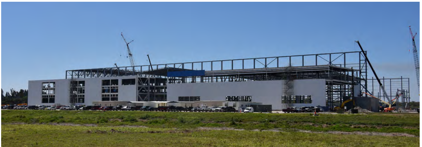
Below: Blue Origin's New Glenn rocket assembly plant under construction.
