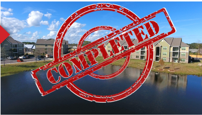
Certificates of occupancy have been issued for all 216 apartment units at Solamere Grand.
