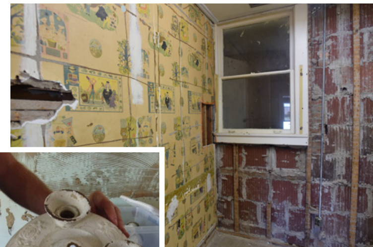
Above: Original wallpaper and terracotta walls inside the old Titusville Bank building.
