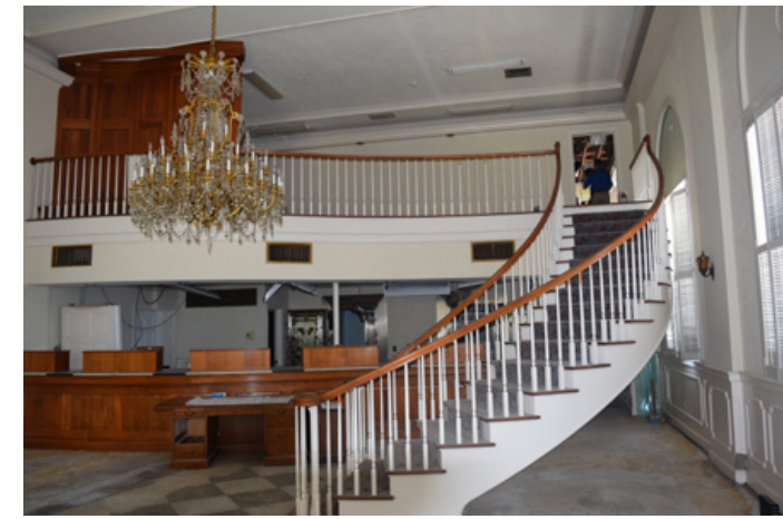
Inside the old bank building, the curved staircase and period chandelier will be preserved in place, while the old bank teller desks behind will be removed. The original bank vaults will also remain.
