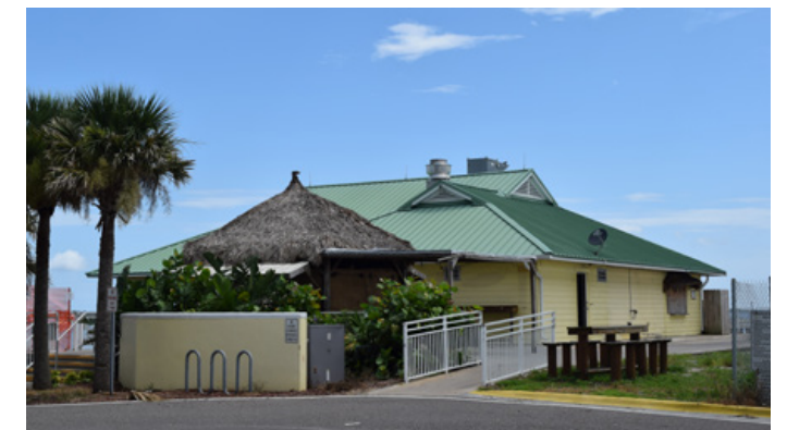
The former Crackerjacks restaurant building and the existing tiki bar that will be torn down and replaced.
