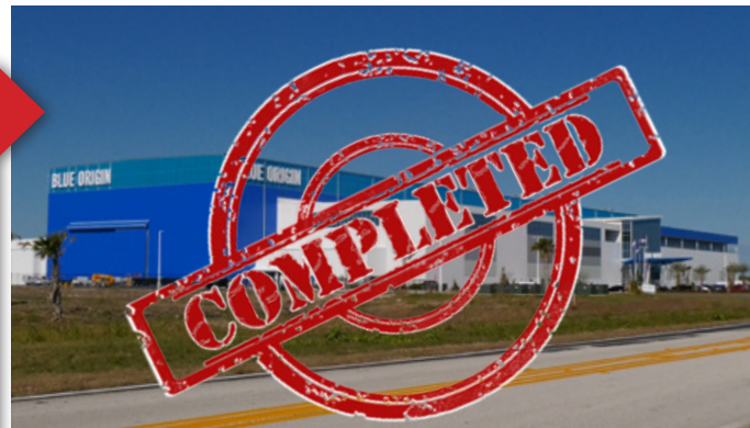
The business office area of the 750,000 sq. ft. New Glenn rocket factory building is complete and occupied.
