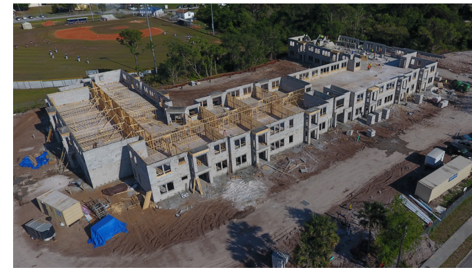
Construction continues on an 84-unit, 3-story apartment complex located at the southeast corner of Sycamore Street and DeLeon Avenue.
