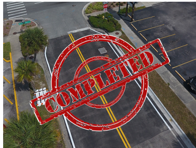
The baffle box located on Palmetto Street in front of Titusville Fire Department's headquarters and City Hall is now complete and traffic through the area has been restored.
