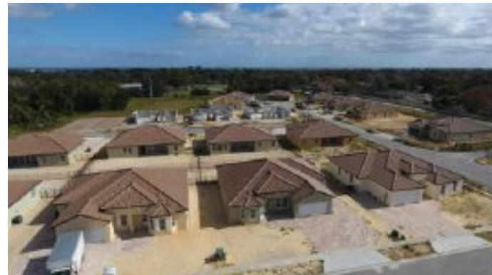
Several new homes are nearing completion in this new residential neighborhood being constructed just west of LaCita Country Club, on Country Club Blvd.
