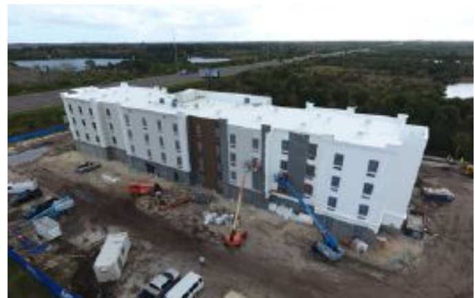
Exterior surface coatings and paint are being added to the walls of the new 124-room, four-story hotel located at the southern-most end of Helen Hauser Blvd, off of SR 50, just west of I-95.
