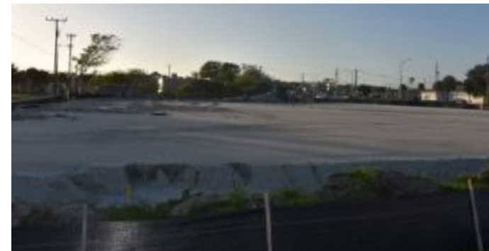
Site work continues for a 16,800 square foot commercial plaza that includes a retail store, restaurant and second floor open air tiki bar and observation deck located at the southwest corner of Garden Street and Indian River Avenue.
