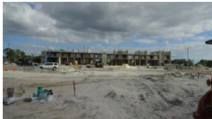
Crews are busily constructing the first floor and surrounding ground work for a new 152-room, five-story hotel, located on the grounds of the former U.S. Astronaut Hall of Fame.
