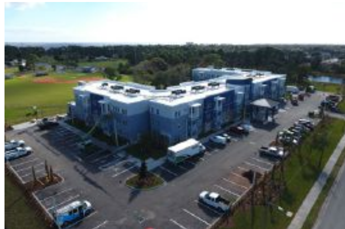
Construction is nearing completion on the 84-unit, three-story apartment complex located at Deleon Avenue and Sycamore Street.
