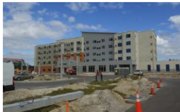
Work is nearly complete on the new Hyatt Hotel, located adjacent to the Boeing complex on south US 1, at Riverfront Center Blvd. The new hotel will consist of 119 rooms, a two-story office and retail building, and an observation deck to view launches from.
