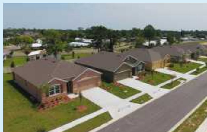
As of July 2021, construction is complete on all 133 lots.
