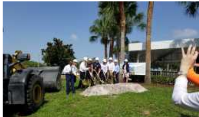
Work began on Courtyard by Marriott, a 152-room, five story hotel with an open deck on the roof at 6225 Riverfront Center Blvd.
