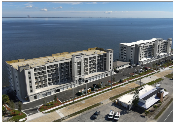
Site and building construction are complete for one condominium building, and site and building construction is nearing completion for the remaining condominium building. The project is located at 1805 Riverside Drive.
