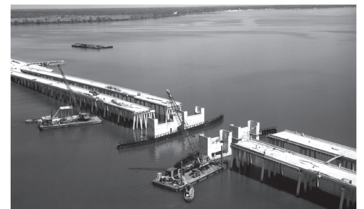
Indian River Bridge under construction in 1964. Photo: NASA
