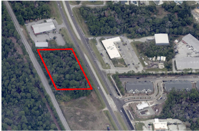
A site plan is under review for a 120,820-square-foot two-story self-storage building.
