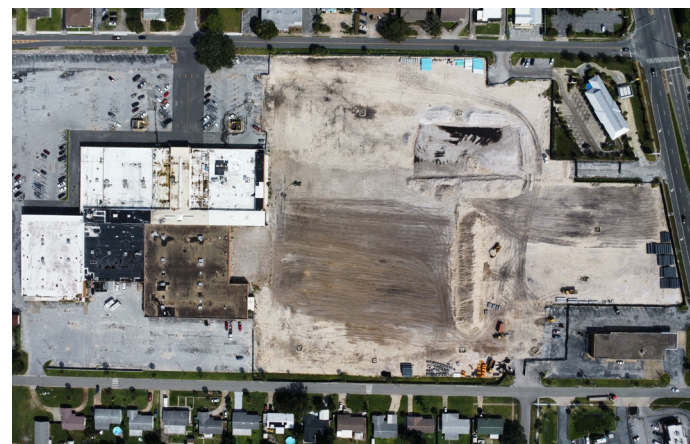
A site permit has been issued for a mixed-use development at the former Searstown Mall at 3550 S. Washington Avenue.
