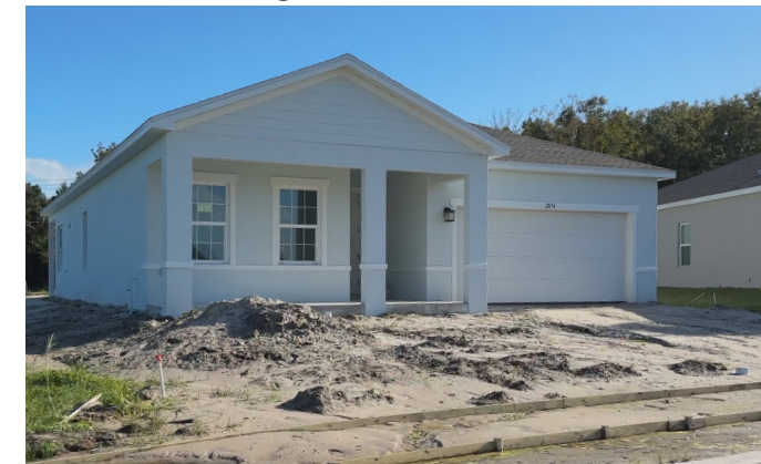
Site construction continues for 143 single-family homes north of Jay Jay Road.
