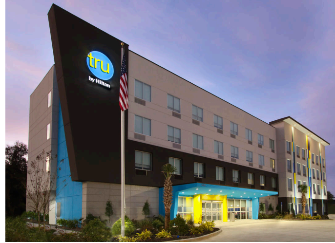
A site plan is under review for a 12,423-square-foot hotel to be located on the north end of Helen Hauser Boulevard.
