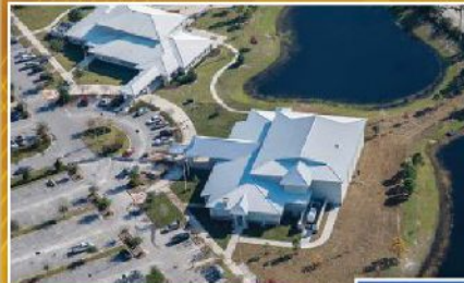
Wickham Park Community Center
