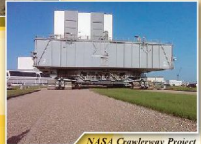
NASA Crawlerway Project
