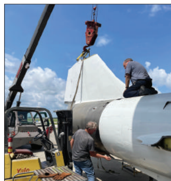
Installing tail cone & vertical stabilizer
